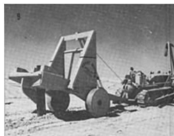
Machines like the GiantRipper with its great steel tooth, were used to rip a trench along the ground in which the pipe was to be buried.
