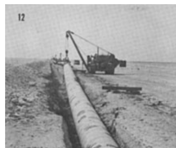
The wrapped pipe was then lowered into the trench and covered over. Sixty per cent of the pipe system was put underground.
