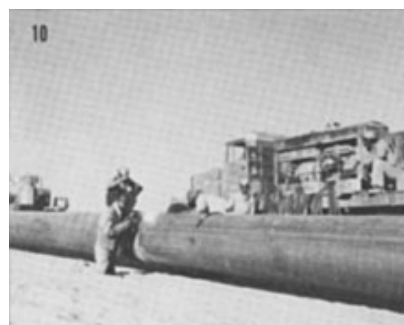
Final welding of the sections fashioned the 93-foot lengths of pipe into one great tube. All told, over 180,000 welds were made on the great line.
