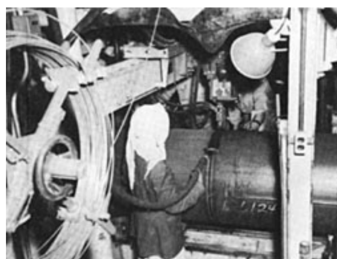
Once on the mainland the 31 foot lengths of pipe were stored in yards. Three lengths were then welded together and these huge 93 foot tubes were ready to be trucked to the construction crews on the desert.
