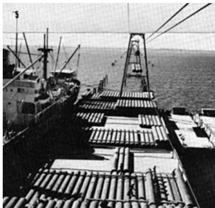
When the pipe arrived at the Persian Gulf port of Ras el Mish'ab, shallow coastal waters prevented ships from getting close to shore. A Skyhook, an ingenious overhead trolley which rode on steel cables strung over towers, took the pipe ashore from a man-made sea-island where the ships unloaded. The Skyhook could shuttle ten-ton loads of pipe to the mainland three miles away in a few minutes.
