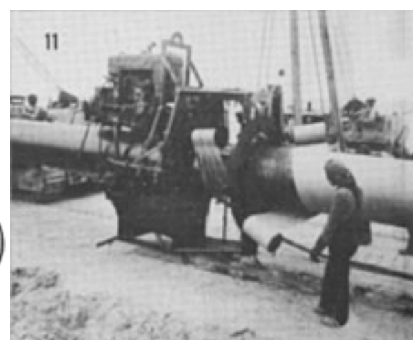
To protect the pipe against corrosion, it was coated with asphalt and machines wrapped it in fiberglass and asbestos felt covering.
