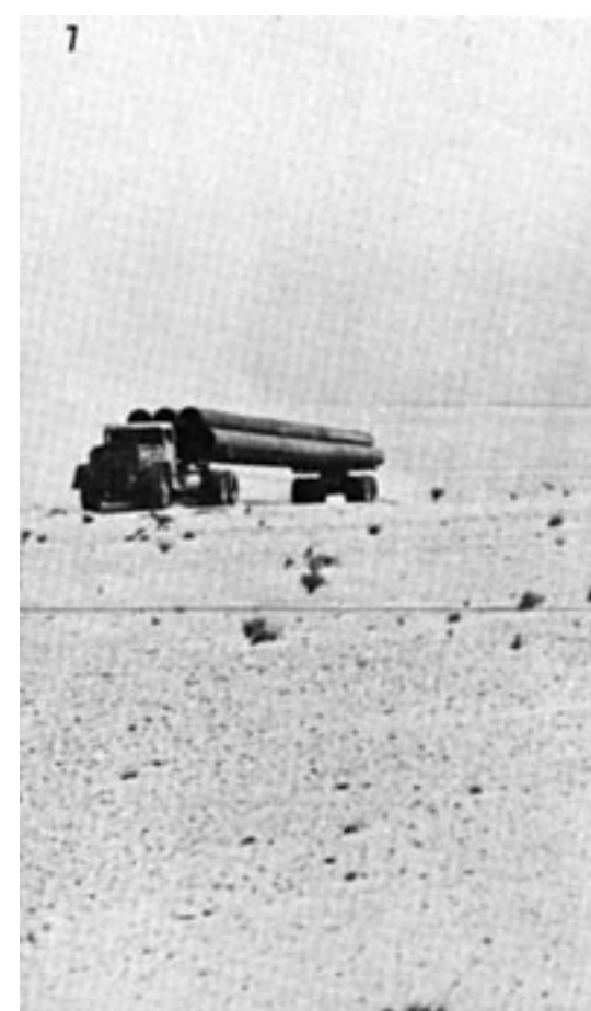
Huge 300 horsepower trucks, equipped with special, low pressure sand tires, hauled the pipe across desert and plain. More than 1500 vehicles made up the desert fleet of cars and trucks that were used on the job.
