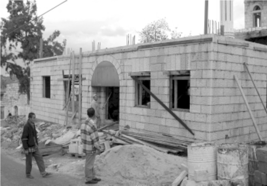
Employment creation in Rantis: Construction of a new health clinic.
